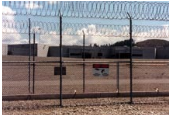
Electrical "Death Fence" Surrounding Pelican Bay
